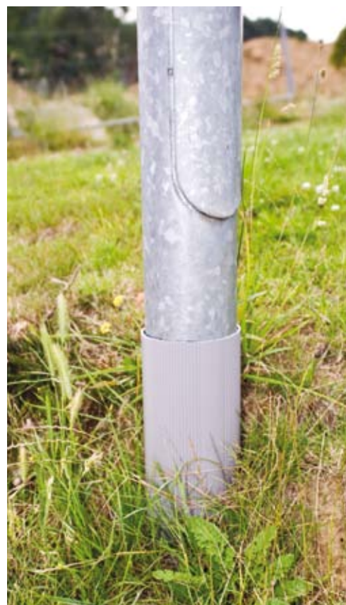
Column protected by strimmex™
