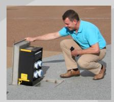
Shown in the background of the photos to the side, is a black Charles Endirect distribution pillar that is used to house the main supply fuses and electrical power meter used to safely supply electrical power to the SIGMA in-ground units.
