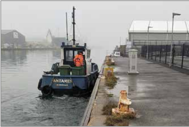
Bespoke, pillar in marine grade 316 stainless steel situated at a ferry port.
