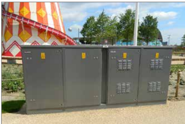
Olympic Park double fronted pillar
