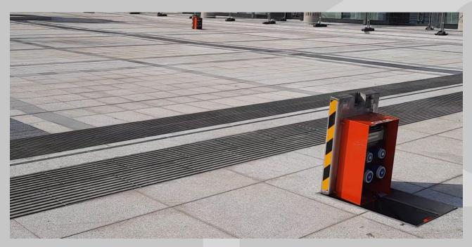
When not in use the GIFAS in-ground unit, with a 12.5T load rating on the lid, blends in perfectly with the surrounding area. Out of site, out of mind, means that it is very unlikely that this equipment can be vandalised in any way
