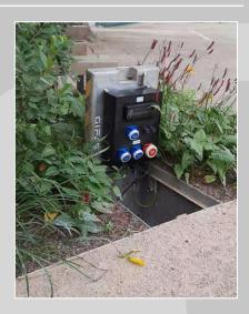
For this project, not only were **GIFAS in-ground units** specified but also a **CEL wall mounted distribution board** complete with electrical sockets and protection was installed in the Main Pavilion to give further access to temporary power for food stalls.
